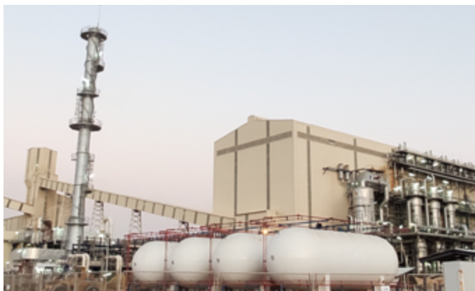
2,500 TPD Standalone Port-Based Sugar Refinery including 12 MW Power Plant with Steam Consumption 0.65 KG/KG R.S.O
