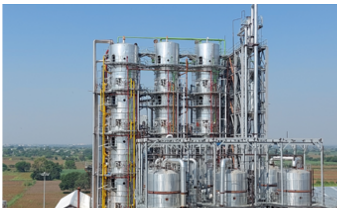
5,000 TCD Sugar Plant – A/B/C Boiling Vertical Continuous Pan (VCP), Design on 29% Steam Consumption
